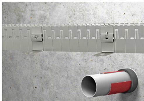
5. Bend two lugs at the end of the metal strap by 90°, connect the other end of the metal strap by inserting the bent lugs into the horizontal slots and bend the lugs back again so that the strap is firmly connected.
